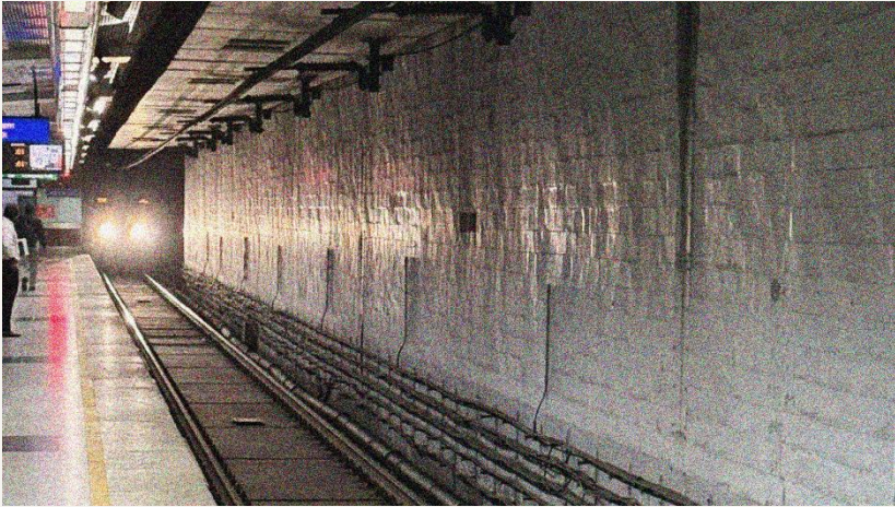
The Delhi Metro is one of the largest metro networks in the world. Photo: Jay Kaushal
